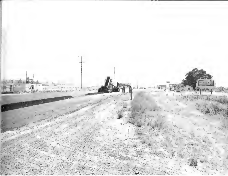
Gap in windrow to control quantity being fed to paving machine
